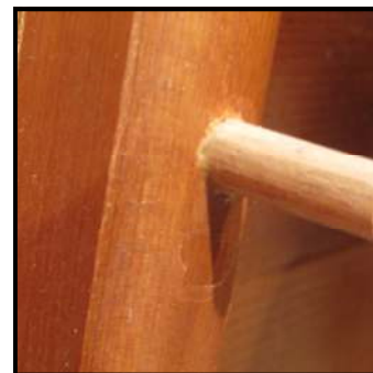
Dowel inserted in place.
