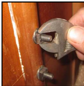
Toggle being tightened
